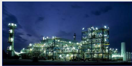
Air Liquide, Port Jerome (SMR +CCS)
