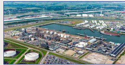
Air Products, Rotterdam (by product H2 from Chlor-alkali process)
